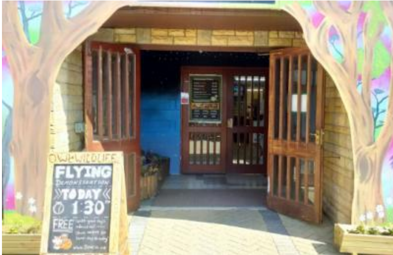
First Set of Main Entrance Doors
