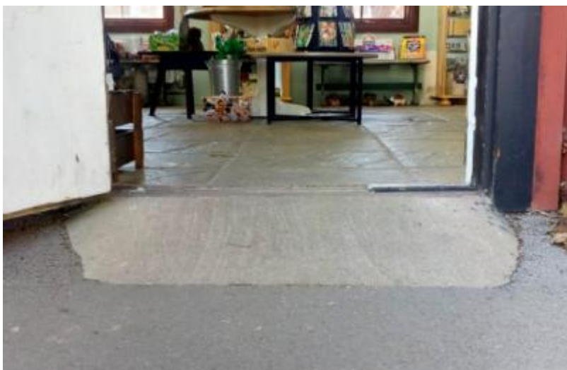
Internal Access Ramp
