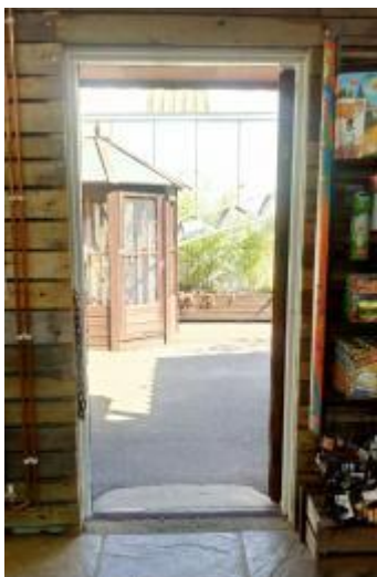
Internal Access Door
