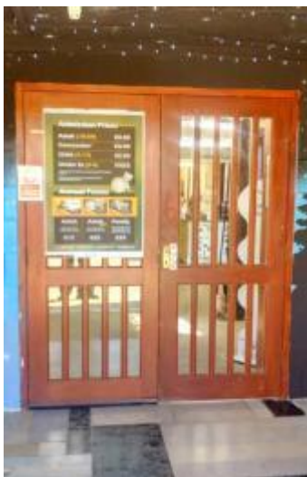
Second Set of Main Entrance Doors
